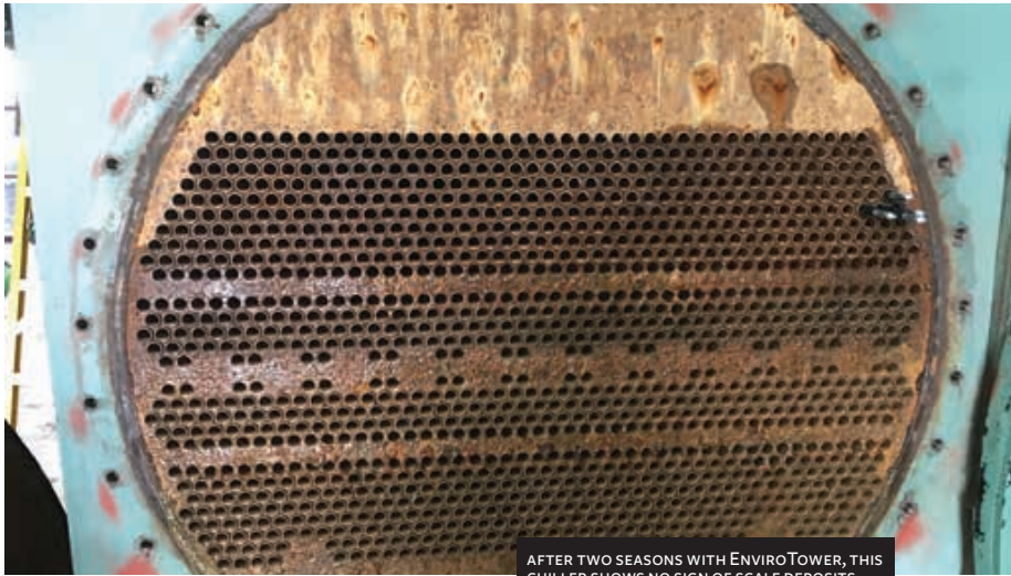
AFTER TWO SEASONS WITH ENVIRO TOWER, THIS CHILLER SHOWS NO SIGN OF SCALE DEPOSITS.
